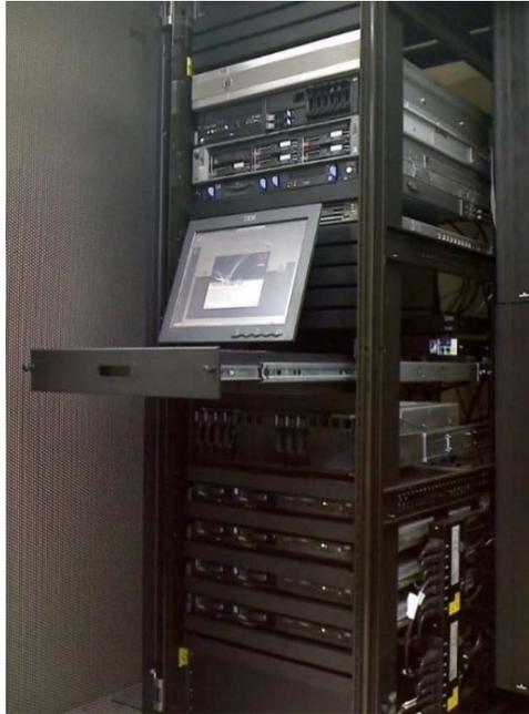
Figure 1.1 – A typical server rack, commonly seen in colocation
